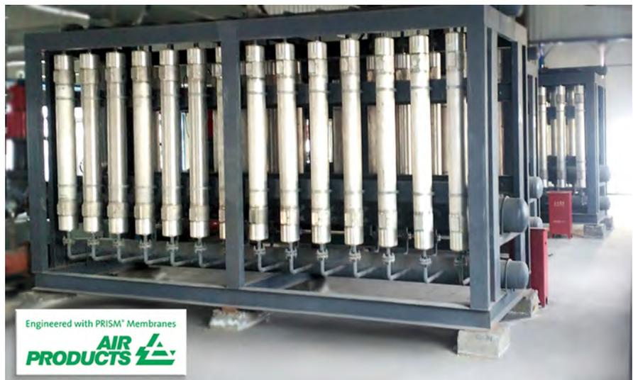
“Using the PB6050 membrane separator makes sense in this processing facility. The low pressure, large gas flow volumes, and economic considerations all made this product and configuration the clear choice to meet all of the customer's requirements.”
